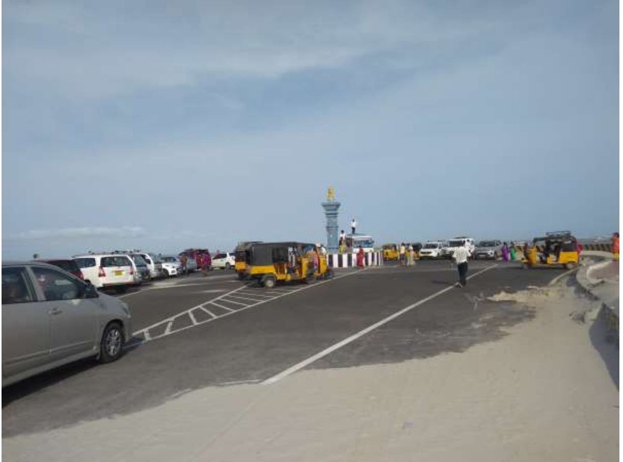
End of the new road at Arichil Munai
