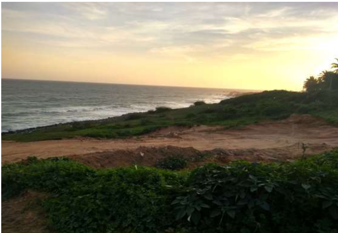
Portion of beach being cleared for promenade
